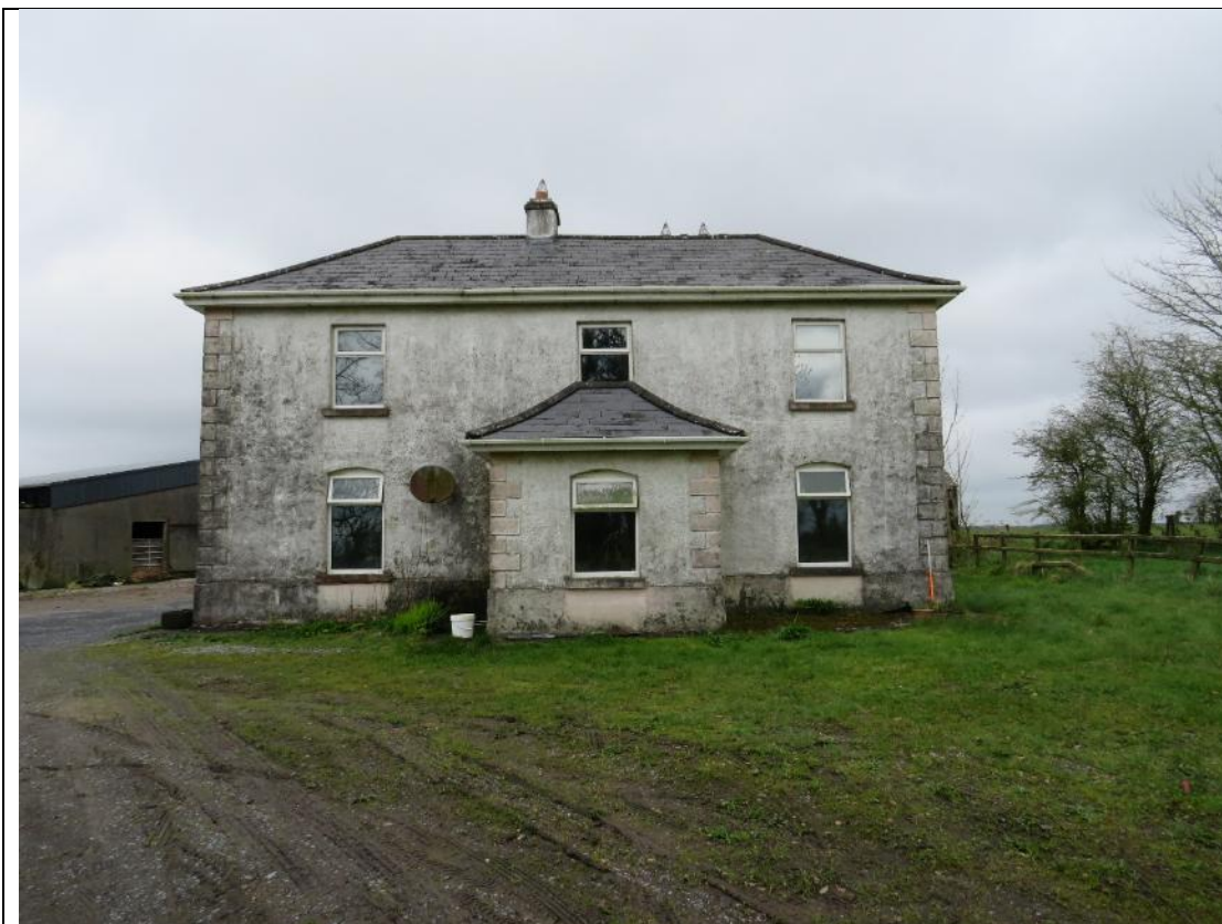
Plate 14-25: Elmhill House (AH91), facing north.
