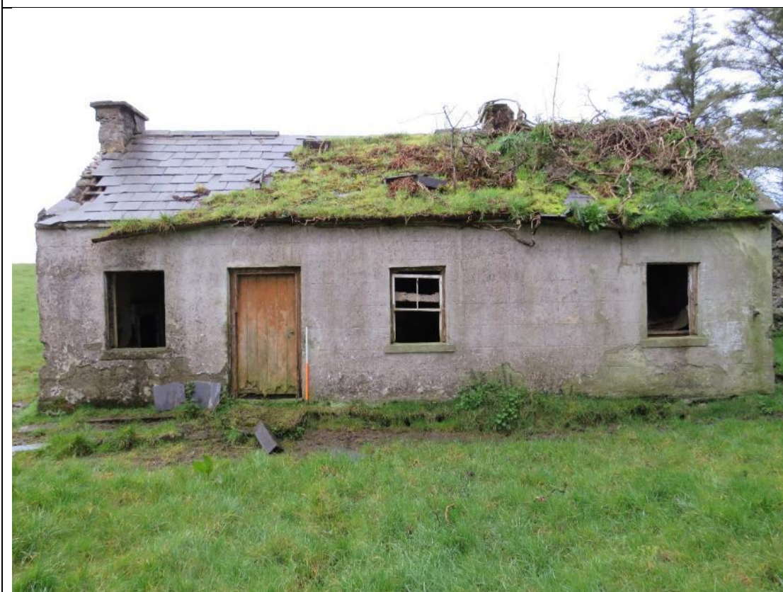
Plate 14-18: Vernacular building CH40, facing north.
