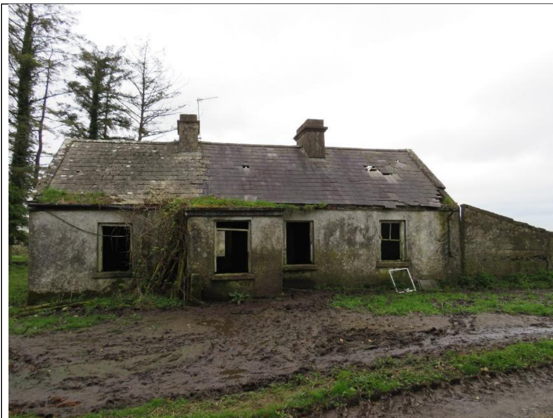
Plate 14-27: Vernacular building CH41, facing west.
