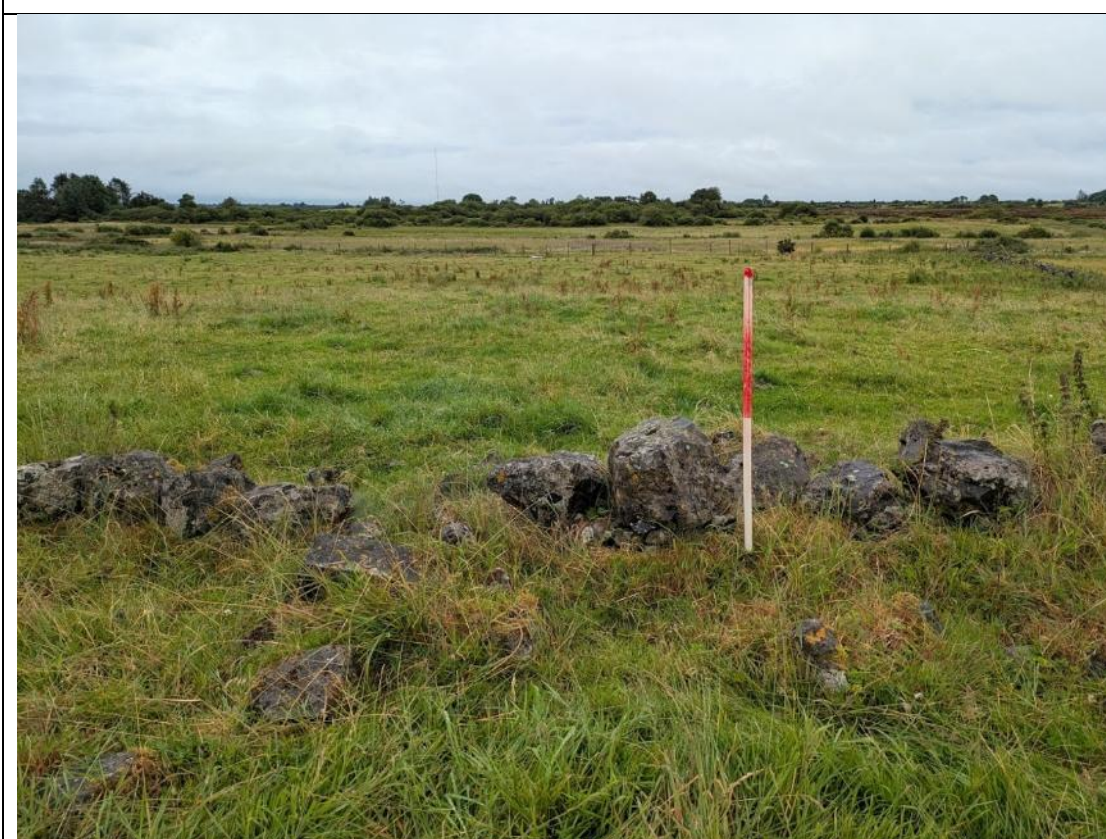
Plate 14-16: Drystone wall (CH58) at location of proposed substation, facing east.
