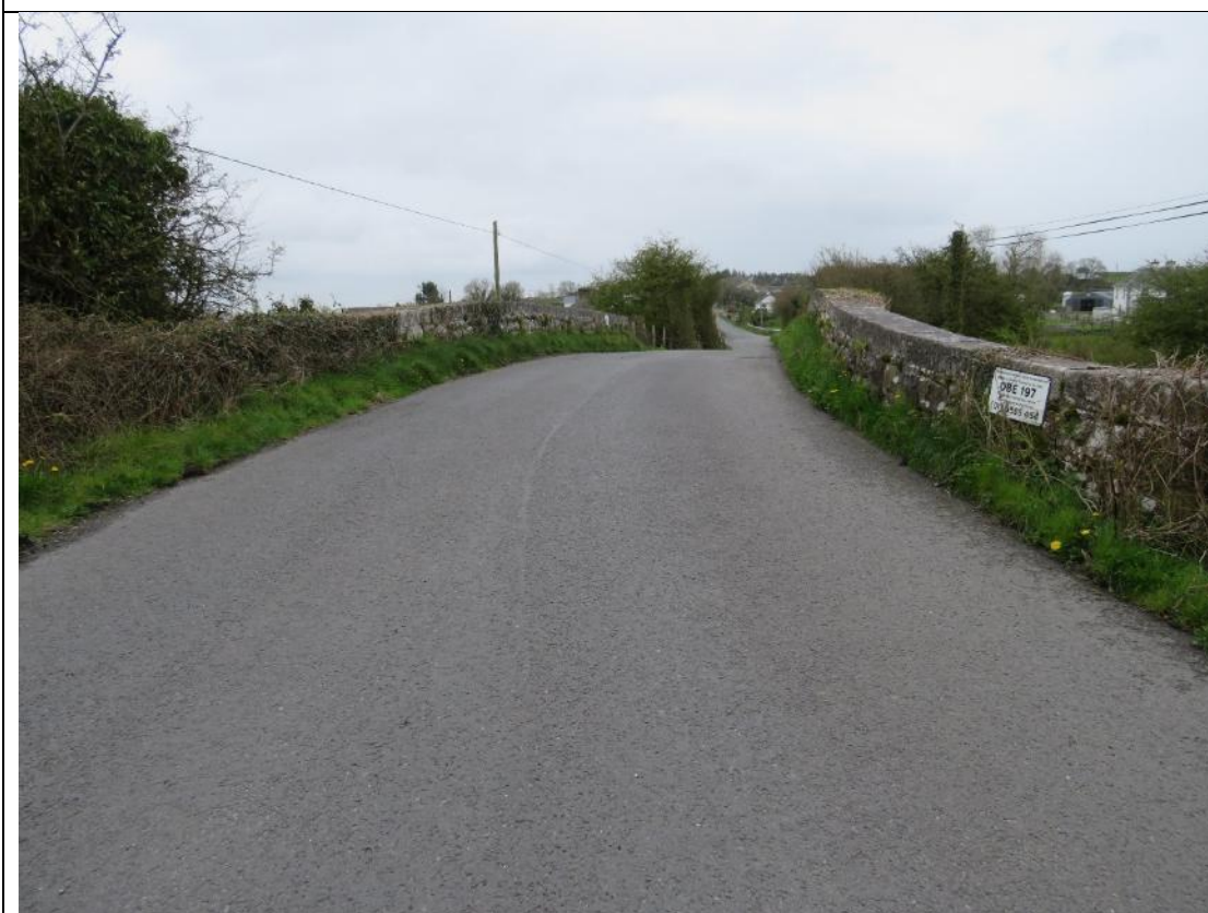
Plate 14-4: Bridge (BH2) over former railway, facing northeast.
