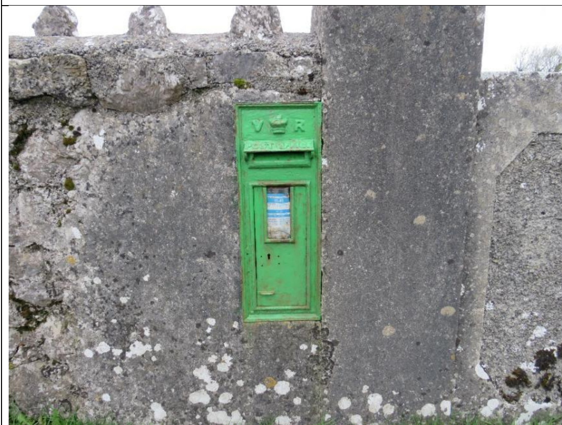
Plate 14-2: Post box (BH4). Facing northwest.
